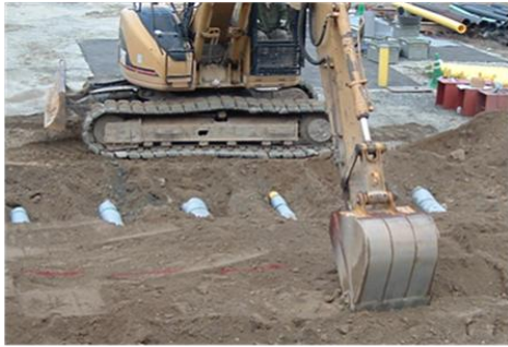
PE pipes with protective sheeting installed
